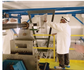
Install new ROC
