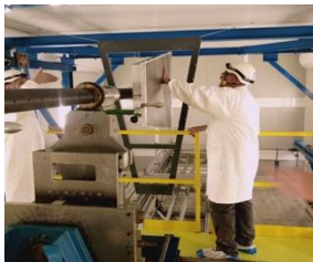
Install new ROC
