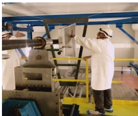
Install new ROC
