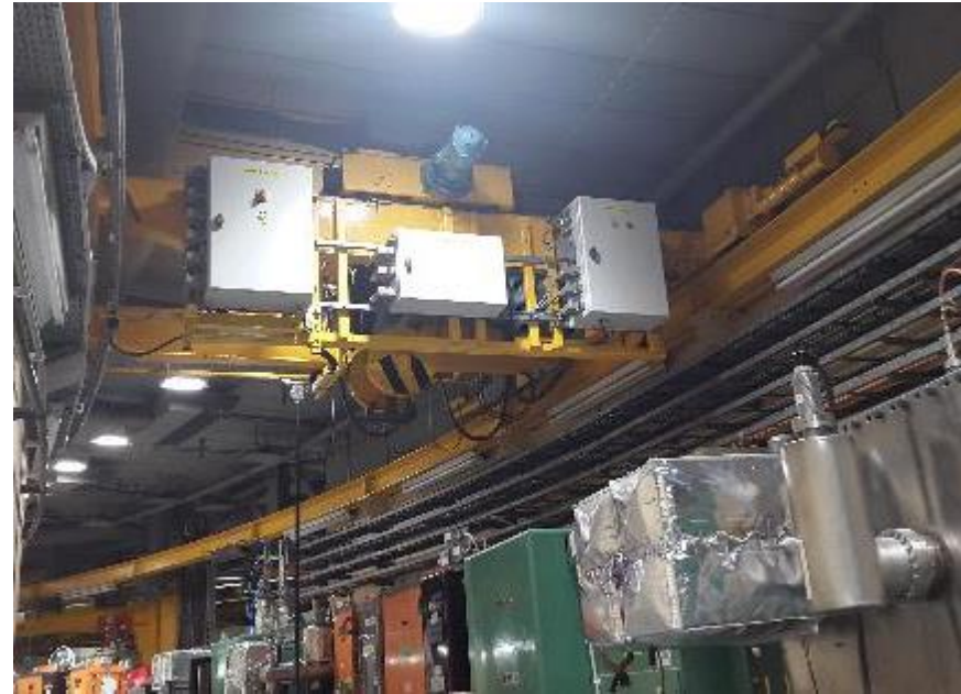
Electrical refurbishment of the three cranes above Booster accelerator
