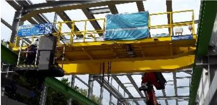
Double girder crane Capacity: 3.2 tonnes Span: 8.360 mm Example of crane «G»
