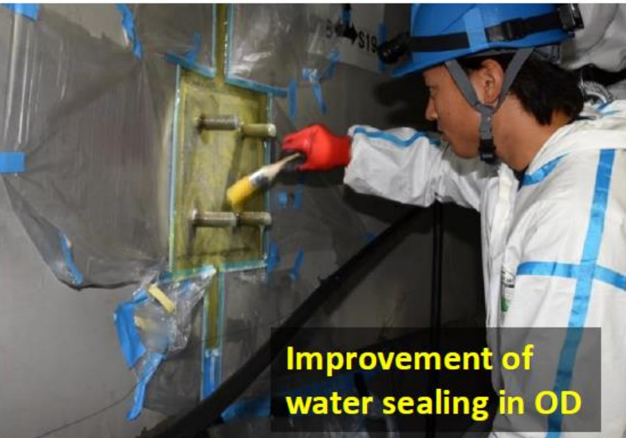
Improvement of water piping in Outer Detector (OD)
