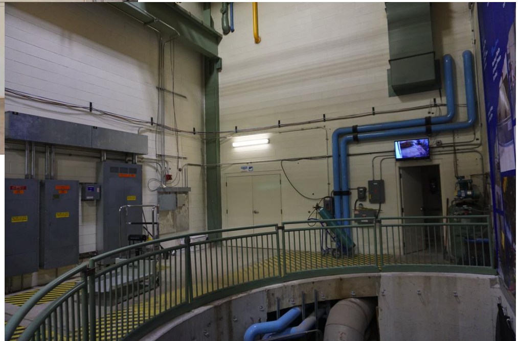
Ground level of MINOS building
