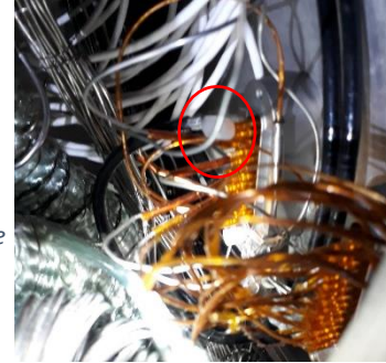
Figure 7: Picture of the LIEBE inside connections for TC and level sensors.
