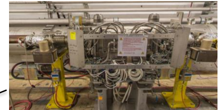
TCLIB: auxiliary protection collimator
