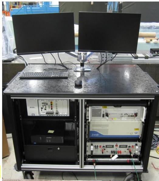
New SSW system
