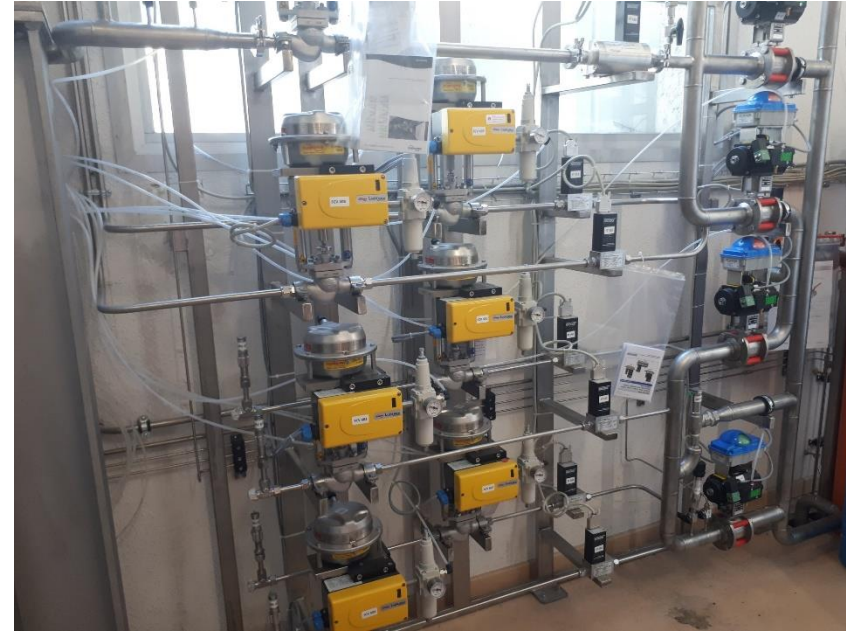
Warm valves + instrumentation manifold made
