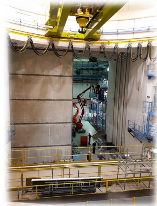
Transmission line installation in ECA5
