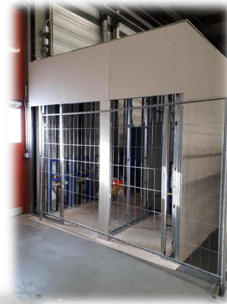
Toilet renovation in BA1
