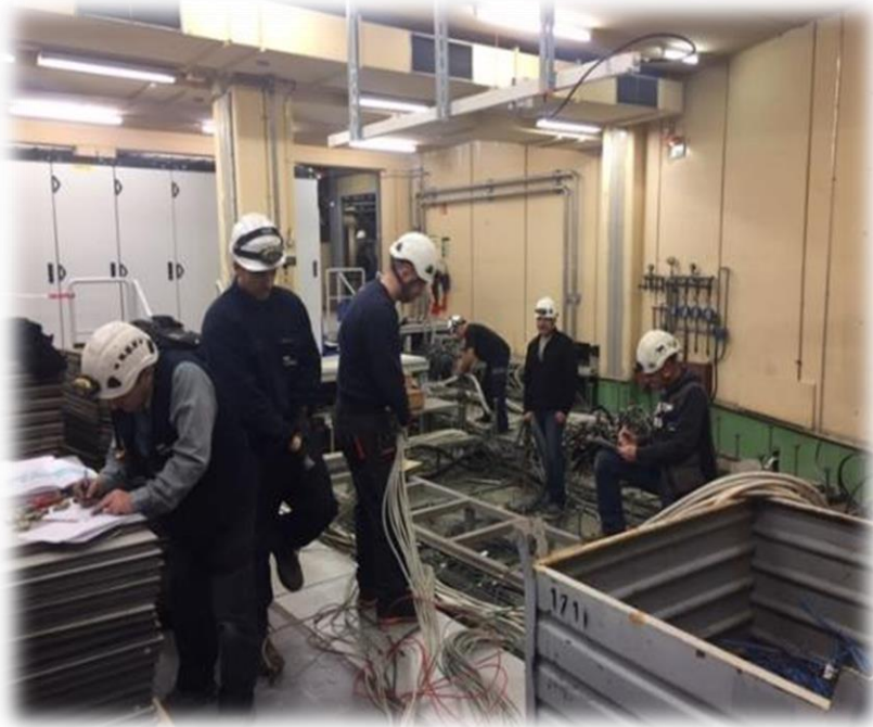
De-cabling, Cabling & Consolidation
