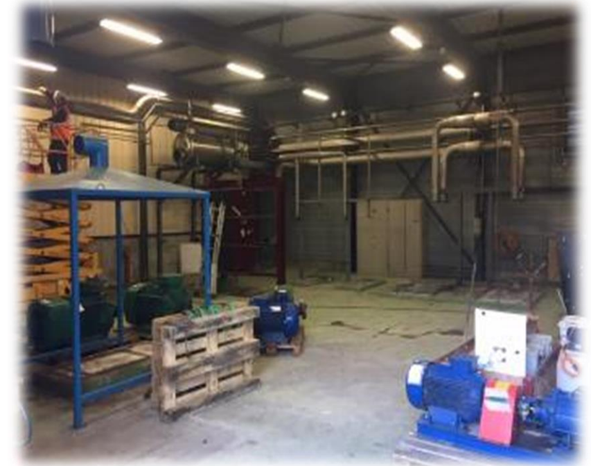
Renovation of the PSB cooling system
