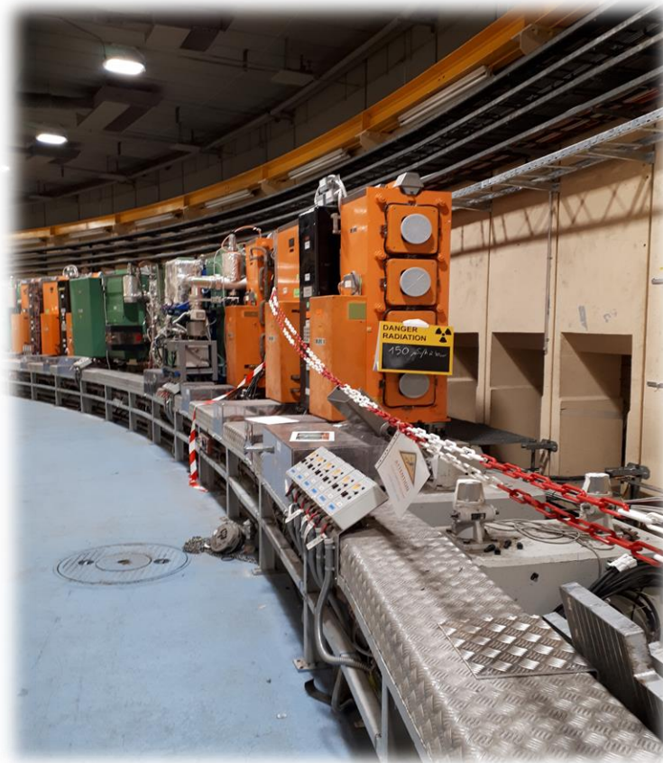
Maintenance & Consolidation of magnets
