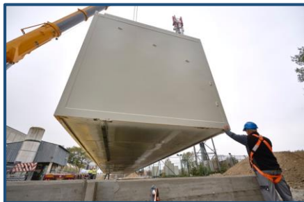
Installation of one of the HLT farm modules
