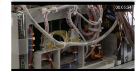
Arm 2 of the LHCf detector in the surface barrack at LHC IP1
