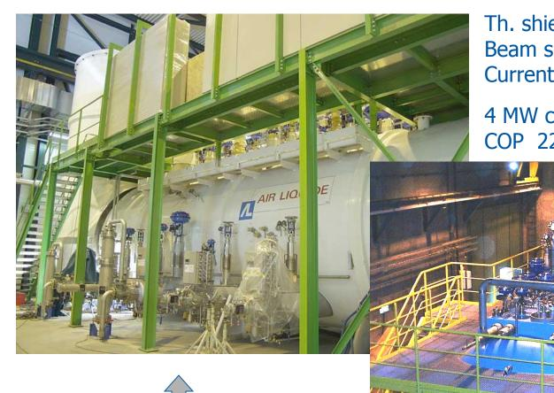
Th. shields: 33 kW @ 50 K to 75 K Beam screen: 23 kW @ 4.6 K to 20 K Current leads: 41 g/s liquefaction
