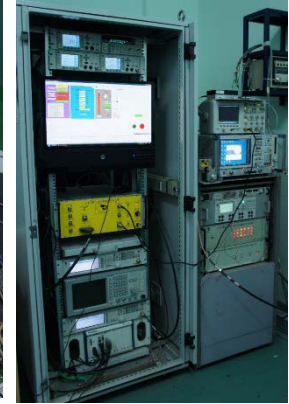
RF System and RF Controls
