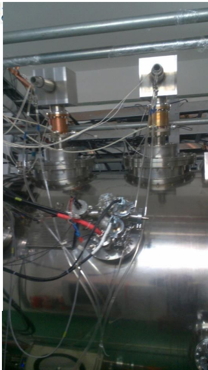
In-cryomodule rf processing of Spোক cavities for TCM of C-ADS Injector-I
