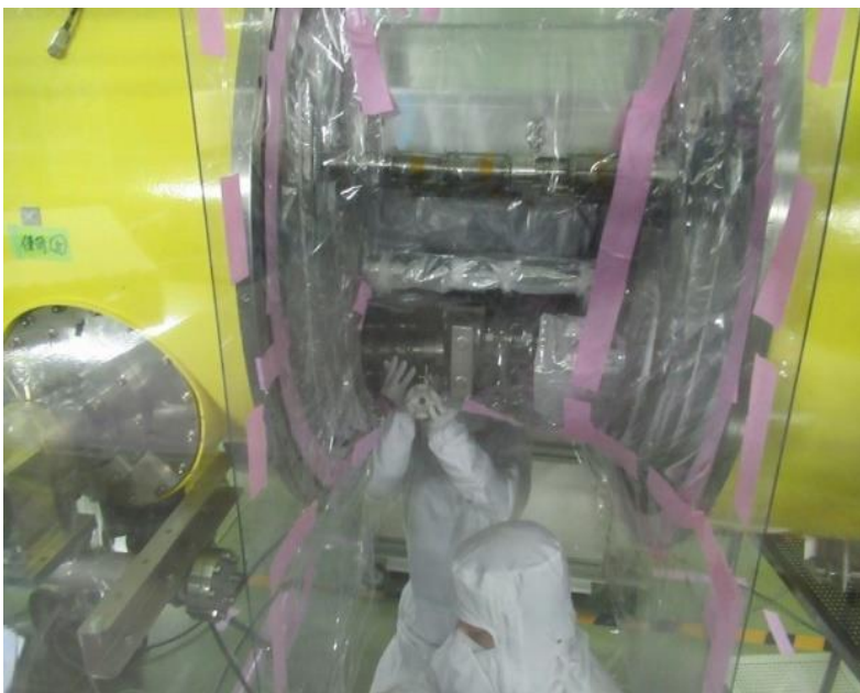
Reconnect the bellows between CM1 and CM2a in KOACH
