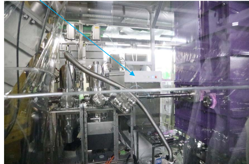
Connection between differential pumping system and CM1
