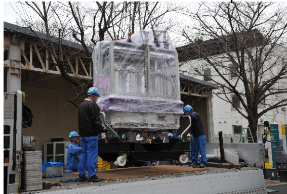
Transport to installation site
