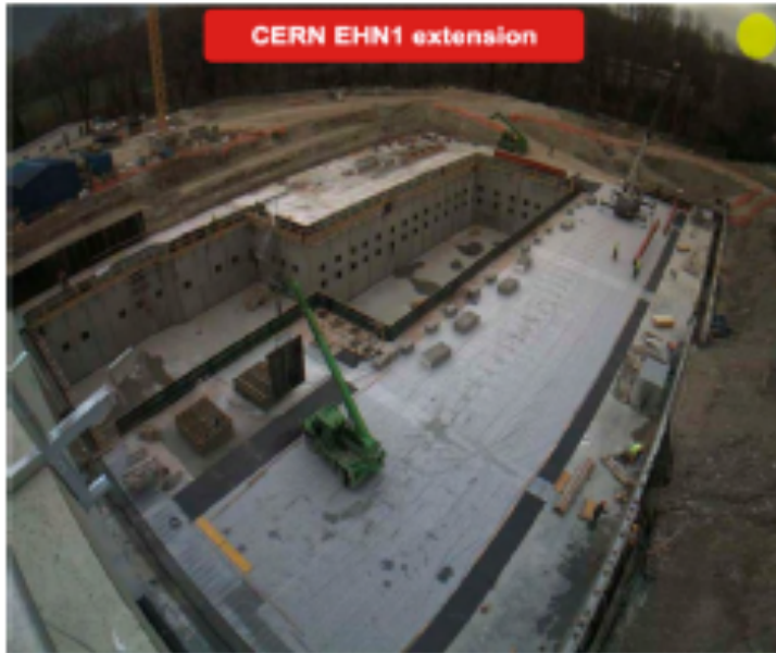
March 2016, construction of EHN1 extension
