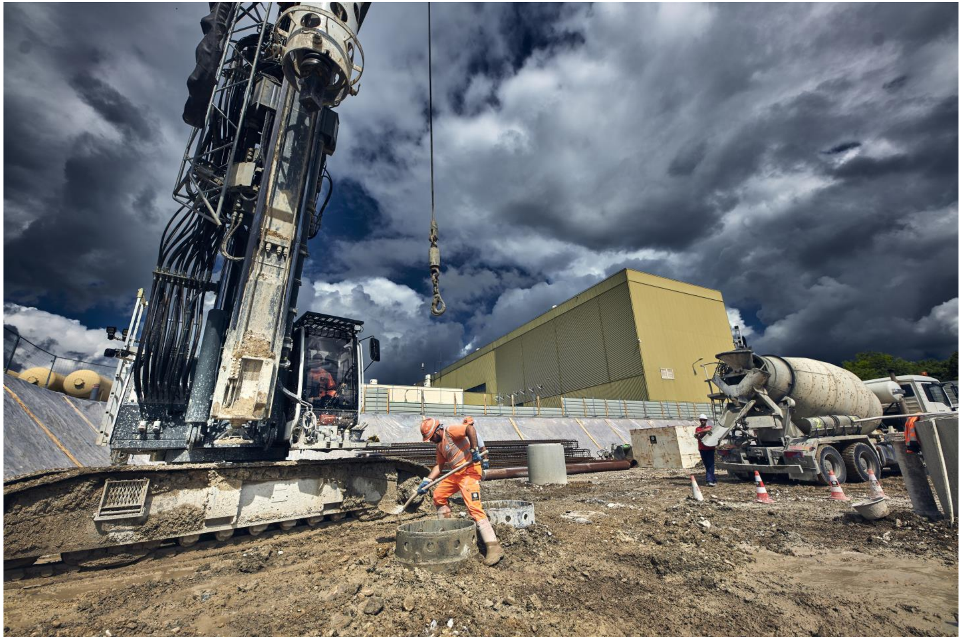
Civil Engineering at points 1 & 5 well underway
