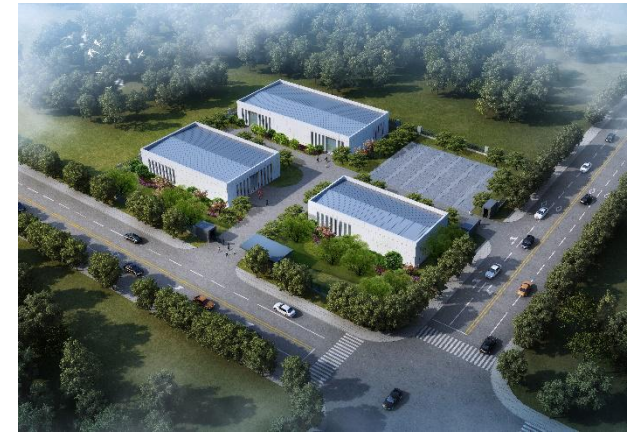
Electric power, cooling and ventilation stations in other places
