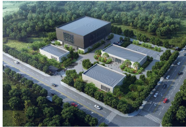
Electric power, cooling and ventilation stations in PA9, PA16, PA23, PA30
