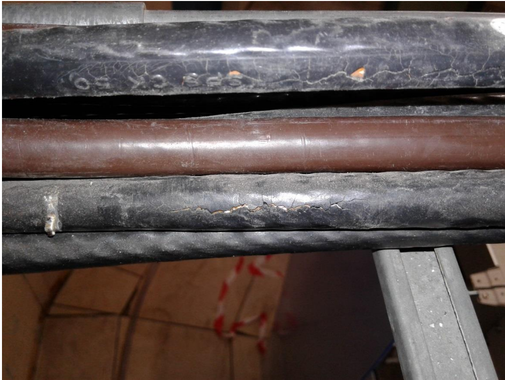
Insulation cracking on a couple of other cables going to R21B.
