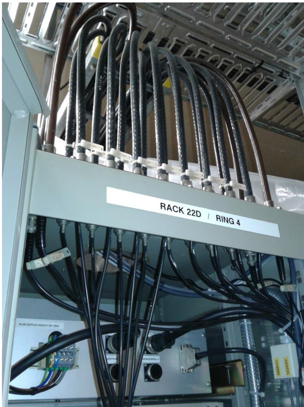
R4 delay cable patch in rack 22D.
