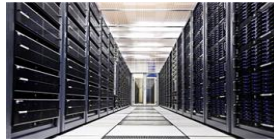
Network and Hardware Controls
