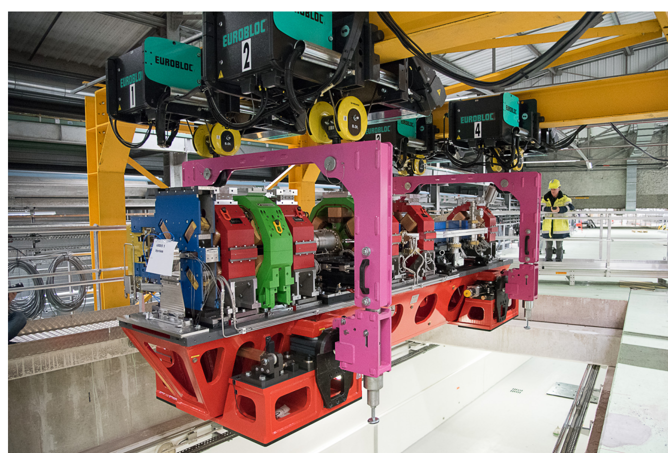
Installation of an EBS girder
