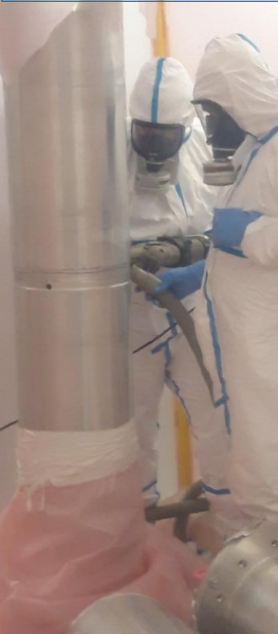
Vertical cutting of low activated part
