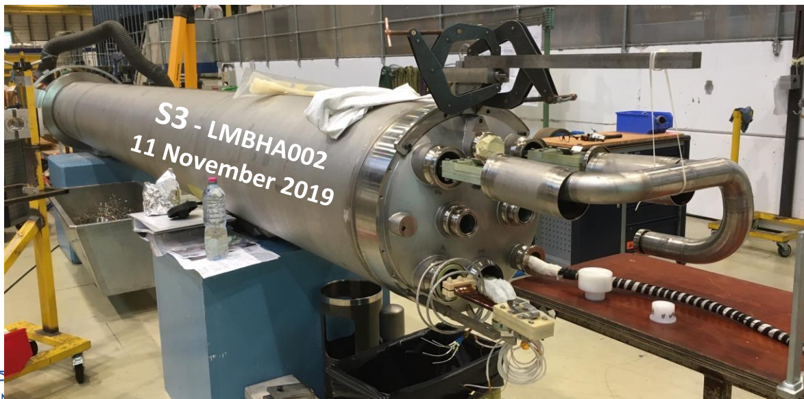
Completion of S3 cold mass ass. y in Bldg.180
