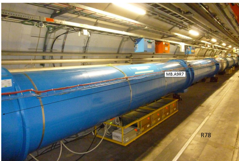
Figure 2 — Picture of area under change, 9R7 at R78 – present MB.A9R7 (18/02/2019)
