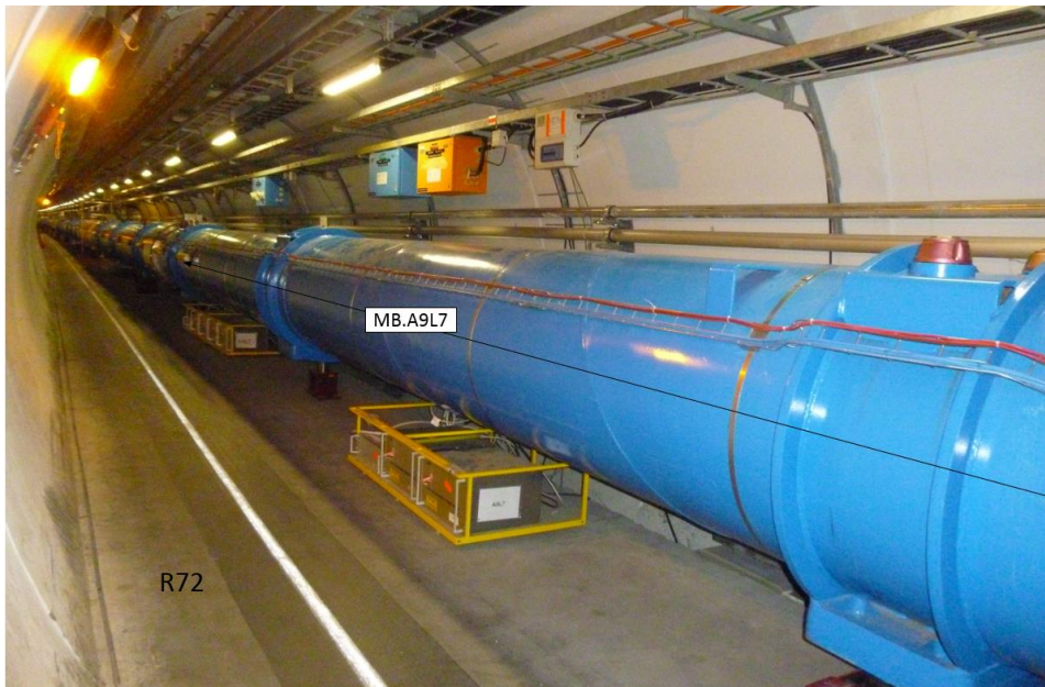
Figure 1 — Picture of area under change, cell 9.L7 at R72 – present MB.B8L7 (18/02/2019)
