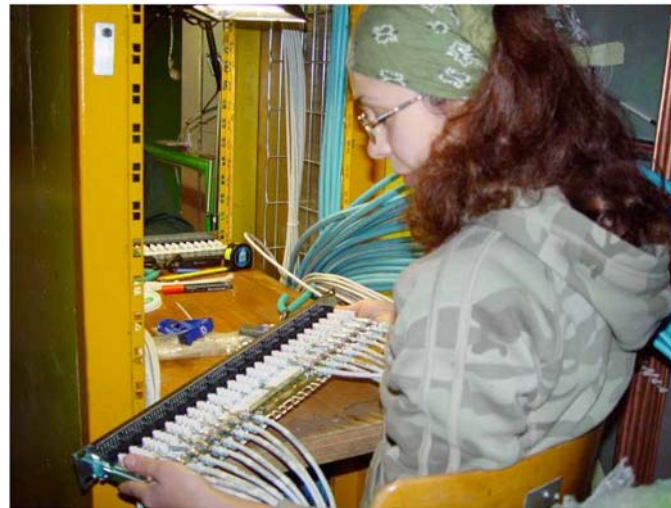
cabling and connector mounting
