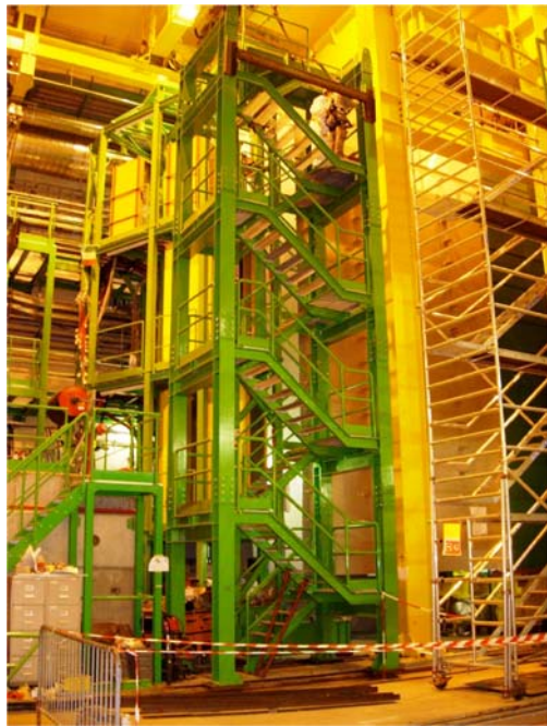
Calo access tower
