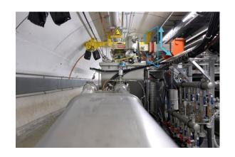
Re-alignment movement tolerance (square bellows):  $\pm$  1 mm in ver/hor (waveguide axis) Today's view: To accommodate more, 1h access BE-RF-PM to free waveguide is required Lab tests will be performed to verify up to  $\pm$  2.5mm.
