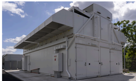
TX-GAIA is housed inside of a new EcoPOD, manufactured by Hewlett Packard Enterprise, at the site of the Lincoln Laboratory Supercomputing Center in Holyoke, Massachusetts. Photo: Glen Cooper.
