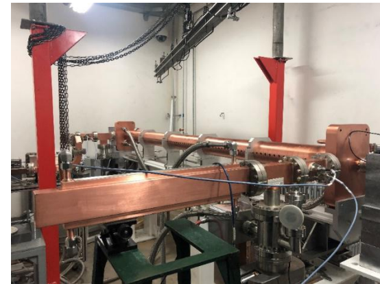
High power test bench
