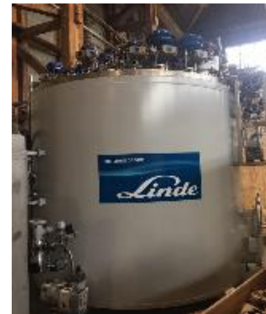
Helium recirculating tanks 2.5KW@4.5K cold box
