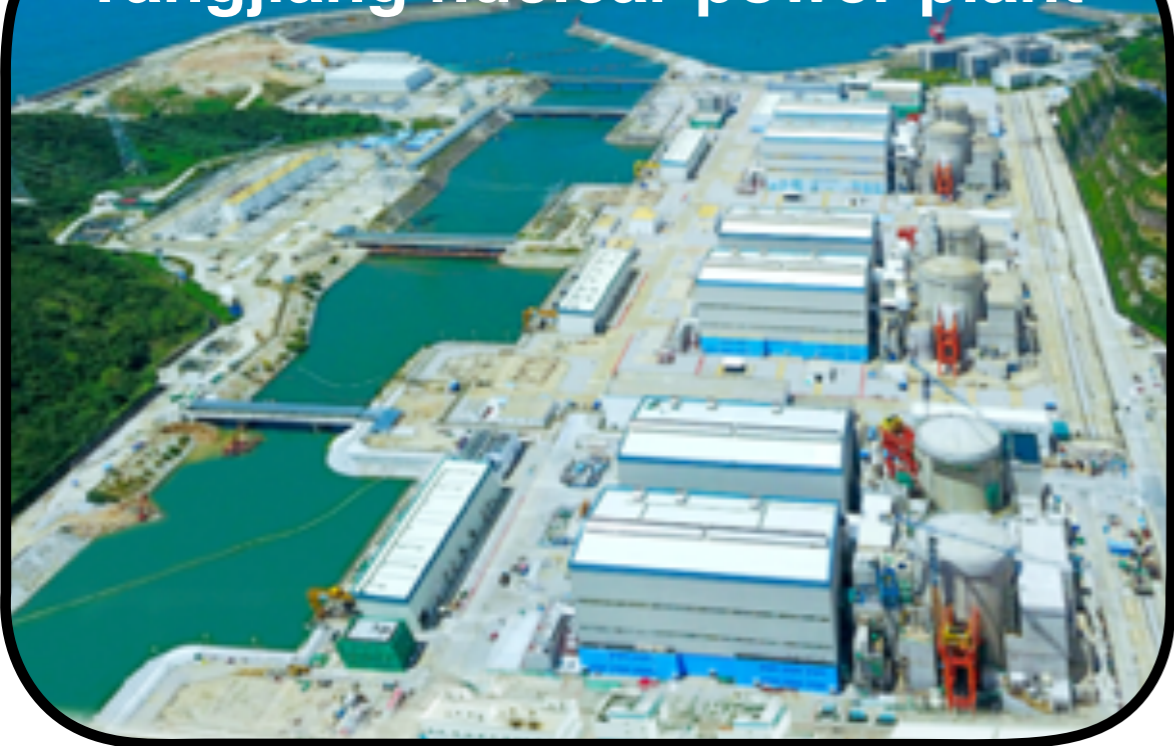
Yangjiang nuclear power plant
