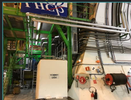
New cooling transfer lines
