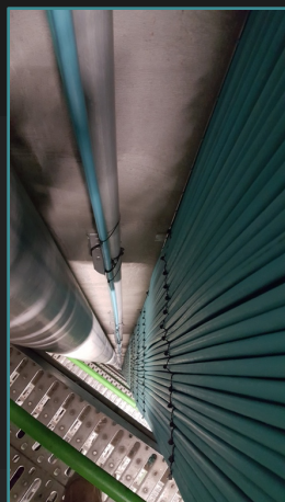
New cooling transfer lines
