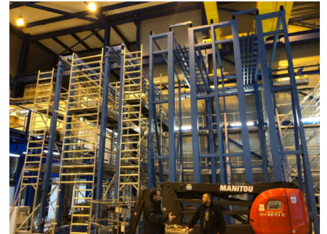
Assembly hall fully prepared
