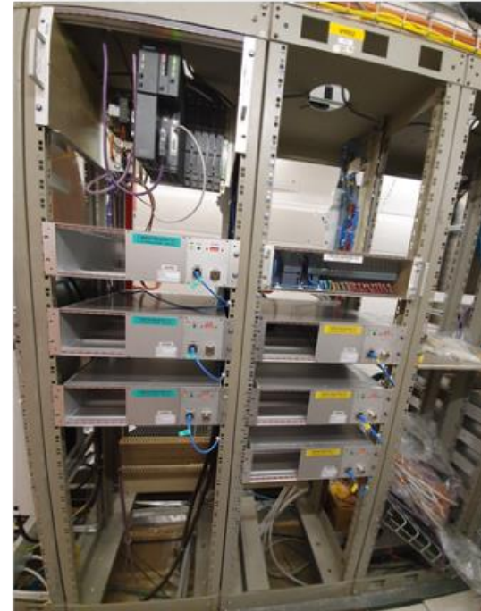
Gauge reading PLC's & controls installation.
