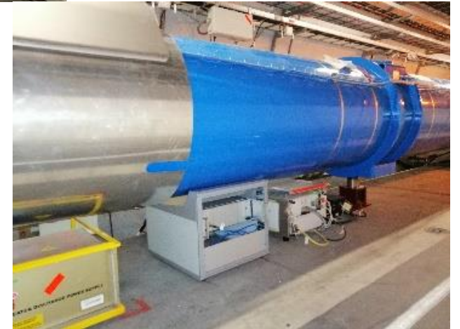
Minirack placed under the magnet with new electronics.
