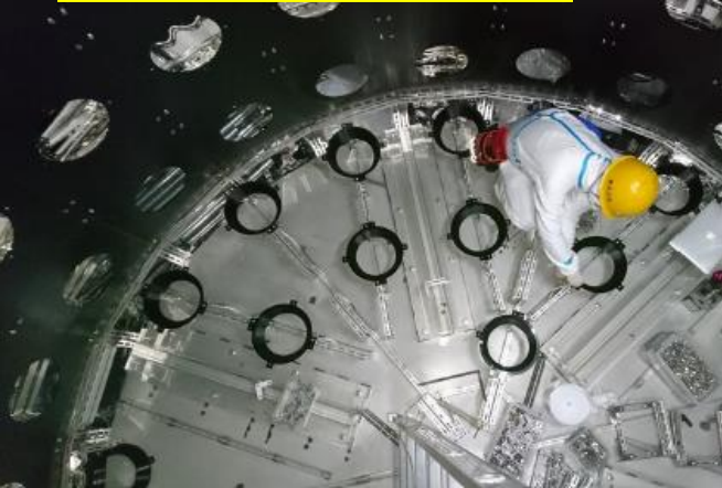
PMT support structure
