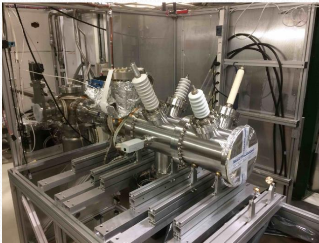
Installed at CERN
