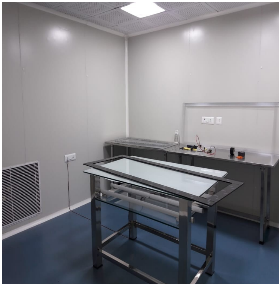
Clean Room Facility
