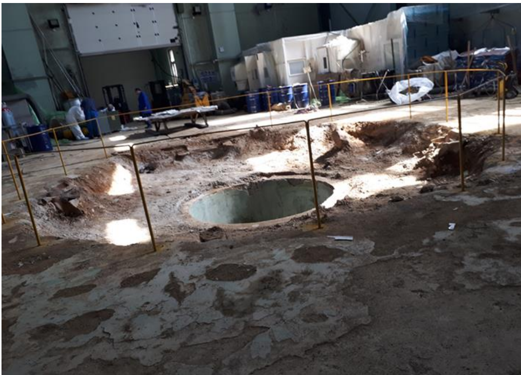
End state of the decommissioning project of the VVR-S Reactor. Reutilization of the building for extension of ELI-NP experimental area. Decommissioning activities for VVR-S reactor were performed with own equipment and workers.
