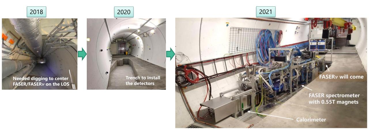
The FASER main detector was successfully installed into the TI12 tunnel in March 2021. Acknowledge great support from many CERN teams involved in the work
