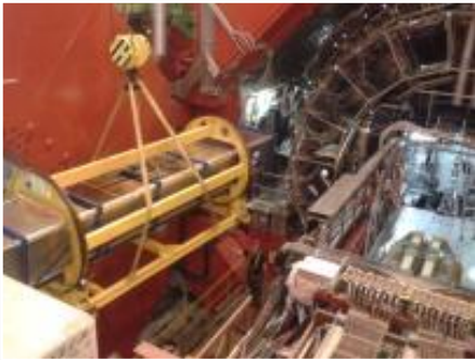
Geometrical infrastructure for detector installation
