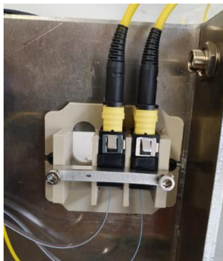
Figure 5: details of the MPO adaptors mounting
