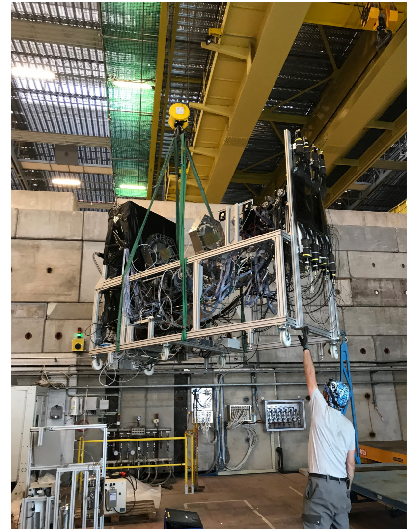
removal of detection system (all components mounted on one frame)
