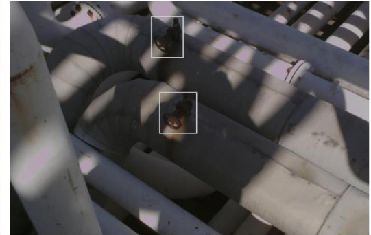
JOINT DEFECTS
