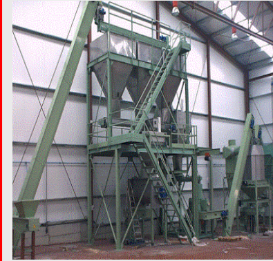
Pilot pelleting plant (300-500 kg/h)
