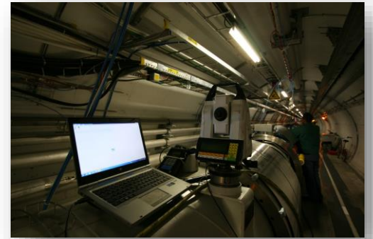
A total station in the LHC
