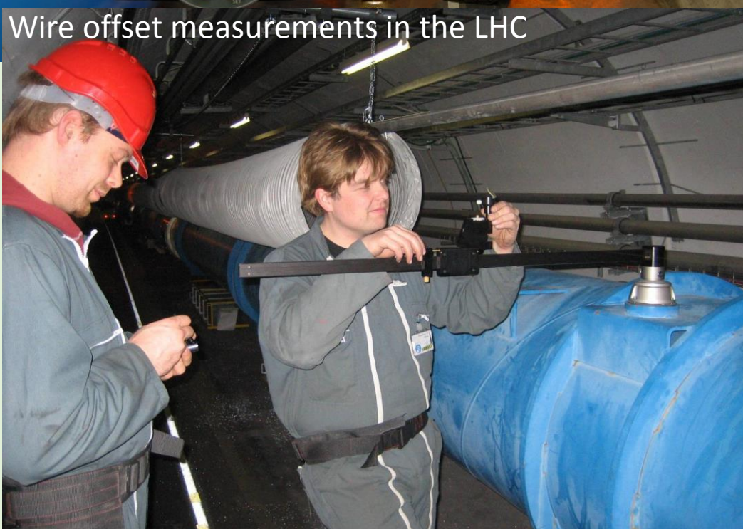
Wire protection pipe
