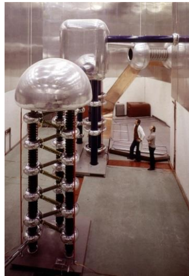
750 kV Cockcroft-Walton Linac2 injector at CERN from 1978 to 1992
