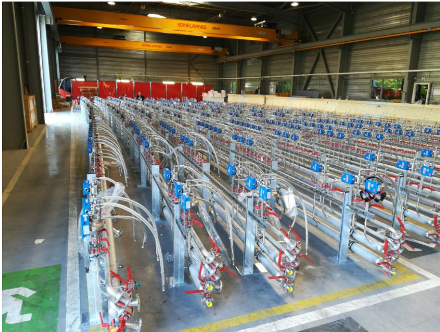
Pipes pre-assembled and tested
