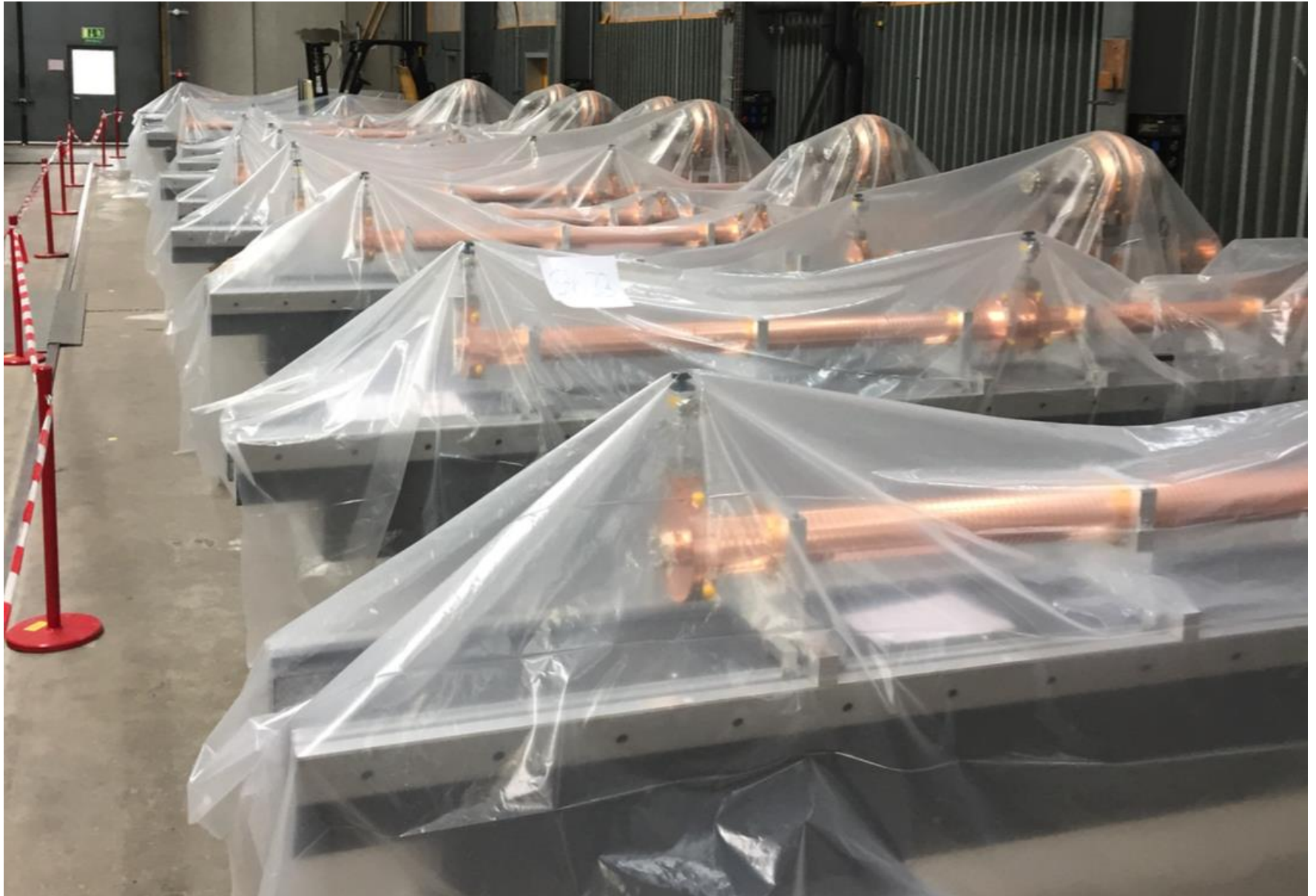
Girders were pre-assembled in a storage hutch
